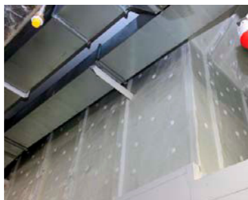
Wall and ceiling insulation – a cutting edge insulation system meeting the highest workmanship standards.
