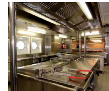
A complete set of kitchen equipment and wall and ceiling surfaces made of stainless steel.
